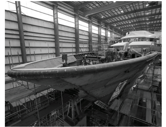
281 foot Cakewalk new construction
